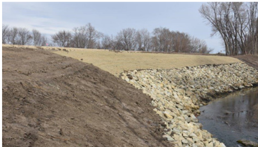
After the EWP exigency streambank stabilization.
